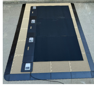
Install the Mats by following the Assembly guide - Assembly of the Mats together . Position the connection cable with the Gateway before proceeding to the next step.
